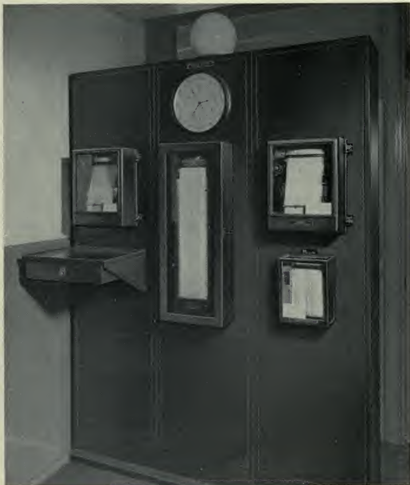
Fig. 30—Clock dial and monitoring equipment associated with the Bell System Frequency Standard, 1937 to date.
